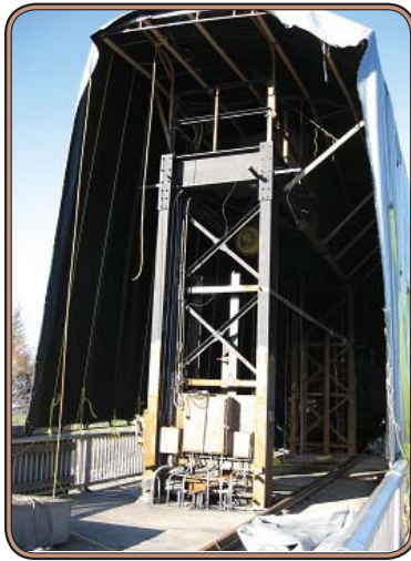
Chesterville dam steel gate.
