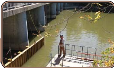
Coffer dam installation.
