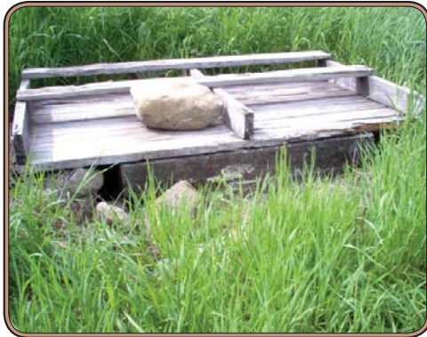
A dug well prior to being decommissioned.
