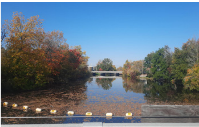
Chesterville Dam, Township of North Dundas
