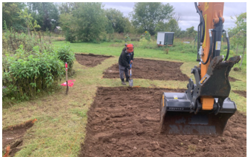
Completion of the Children's Butterfly Garden, Township of Edwardsburgh/Cardinal
