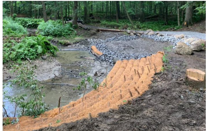
Shoreline restoration, Township of Russell
