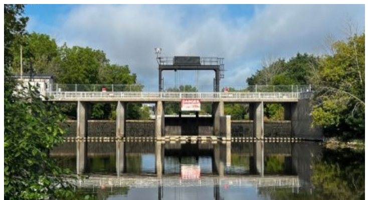
Chesterville Dam, Township of North Dundas
