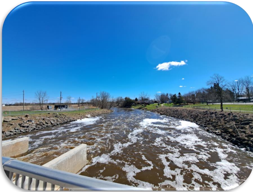
Chesterville Dam, looking downstream (April 16th)
