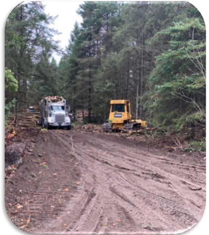
SNC 29 Logging Operation Township of North Glengarry
