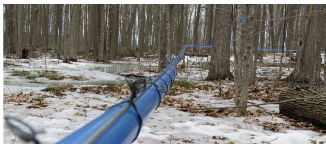
Pipeline through Oschmann Forest in North Dundas
